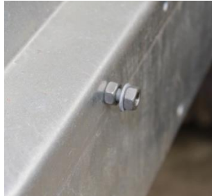
Nuts fitted on outside
