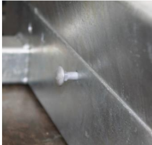
Bolt inserted from inside
