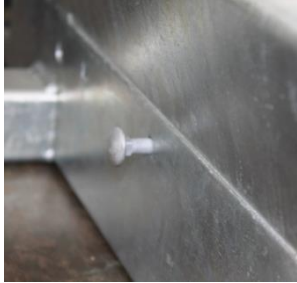
Bolt inserted from inside
