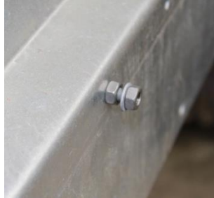
Nuts fitted on outside
