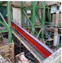
Coveya installed a 20.0m GP750 conveyor which fed the material from the basement floor to the back of the lorry, and was loaded by a 14 ton excavator. The project included;
