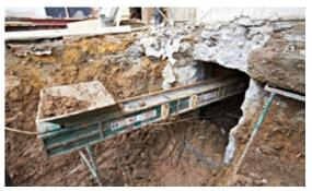
The Easikit<sup>™</sup> 450 is a simple and compact modular system with a large capacity, which is perfect for low volume material handling. Its robust design supports the removal of rubble and light hard core and it also has a detachable feed hopper.
